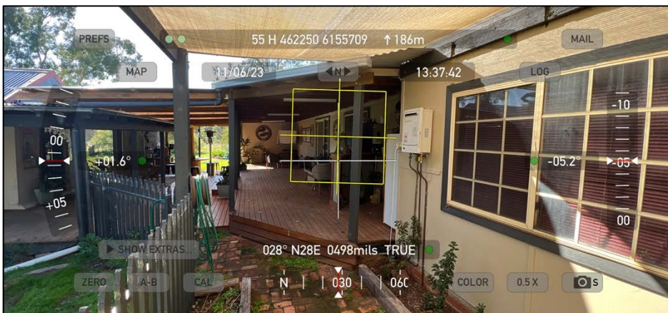
Photo point 6 Showing the general condition of the existing residence.
