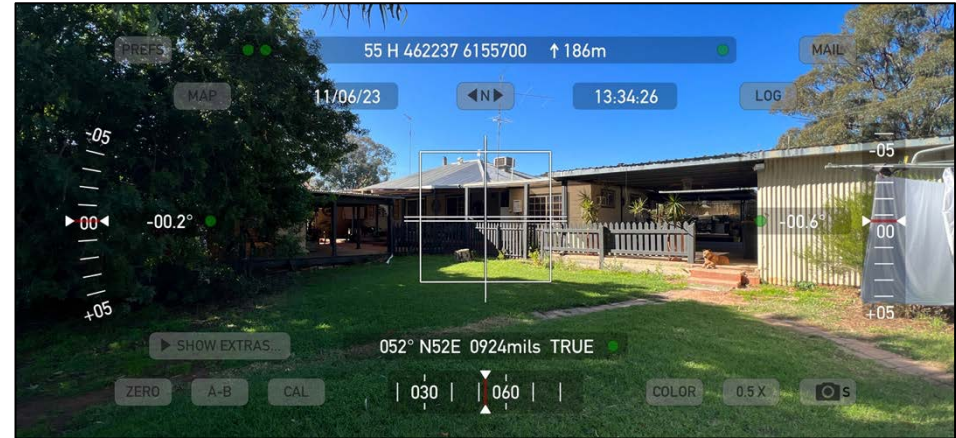
Photo point 7 Showing the established and well-maintained gardens to the southwest of the existing residence.
