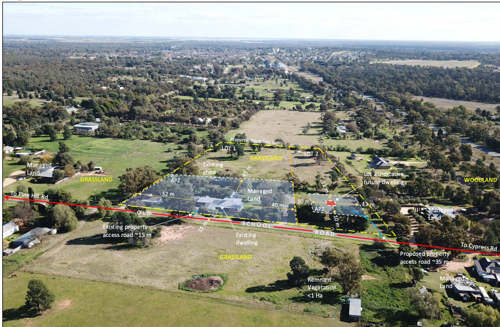
Figure 11 – Aerial overview looking west showing existing residence (Lot 1) APZ, indicative building footprint (Lot 2) APZ, access, and vegetation classification of the site. Indicative only. Not to scale (Hague, 2023)
