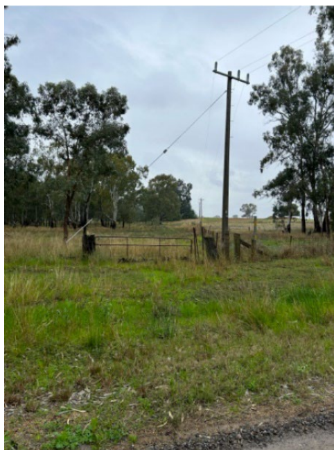
Figure 2 Attached image 24 July 2023
