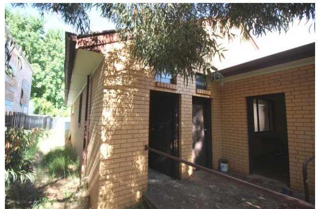
Photo 6: view of former Church & Hall rear area/toilets
