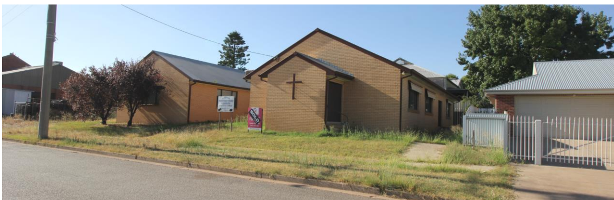
Fig 6: view of the front and east side of the former Church and Hall from 1 Elwin Street
