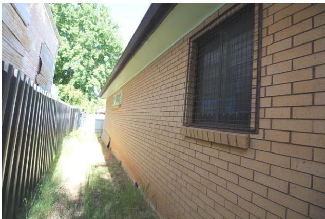
Photo 5: view of former Church – north facade
