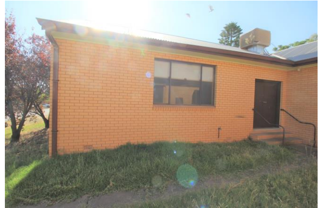
Photo 10: view of former Church Hall – east facade
