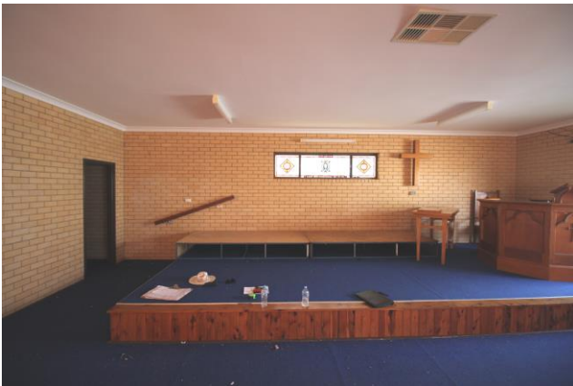
Photo 13: view of former Church – interior
