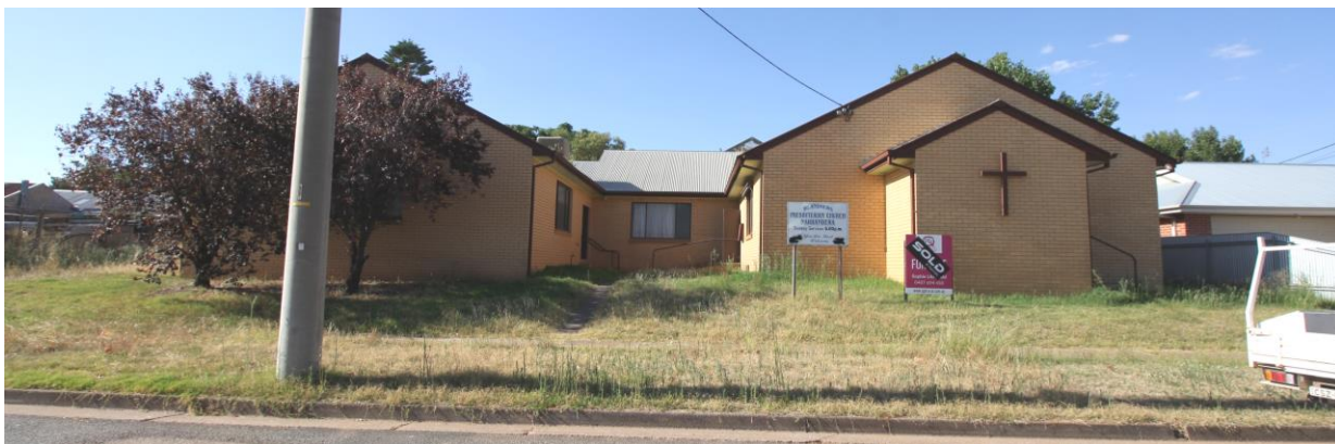
Fig 5: view of the front of the former Church (right) and Hall (left) from Elwin Street
