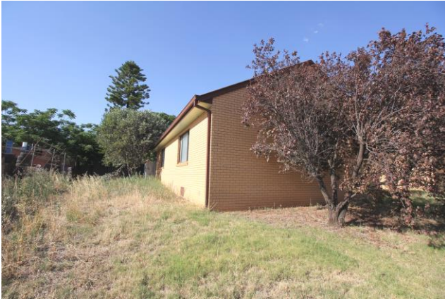
Photo 9: view of former Church Hall – south & west facade
