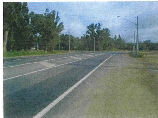
Figure 2.3: Newell Highway (looking west towards the Sturt Highway intersection)
