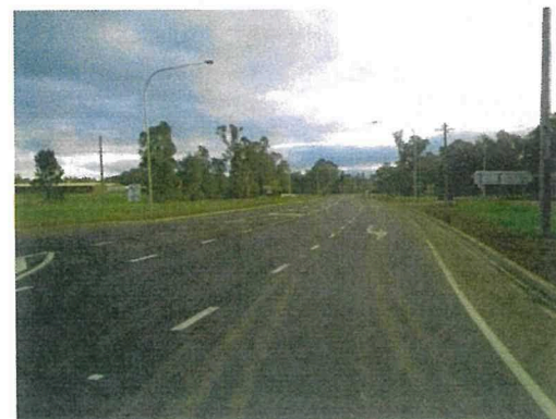
Figure 2.5: Newell Highway (looking west to the site)
