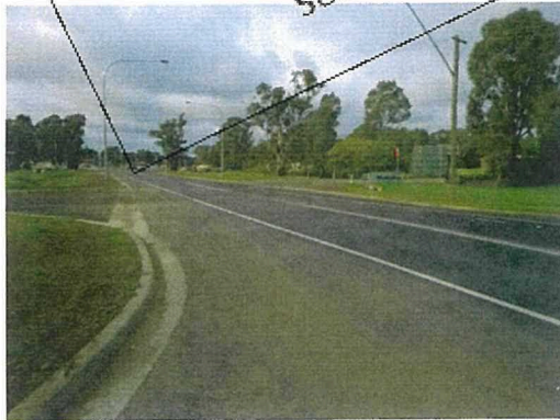
Figure 2.2: Newell Highway (looking east towards the local access road and the site)
